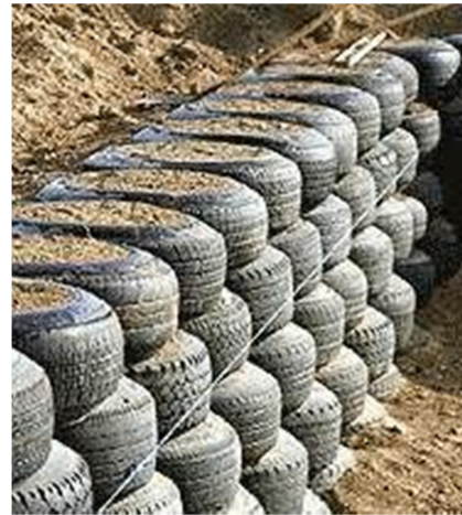
Figure 5: Salvaged tyres used to build retaining walls
