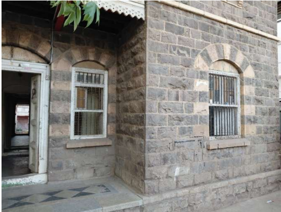
Fig 3 : Shows Stone as a Material
