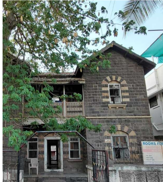
Fig 7 : Shows Gable Roof and recessed window
