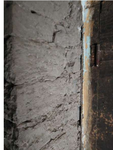
Fig 4 : Shows Lime Mortar and thick wall
